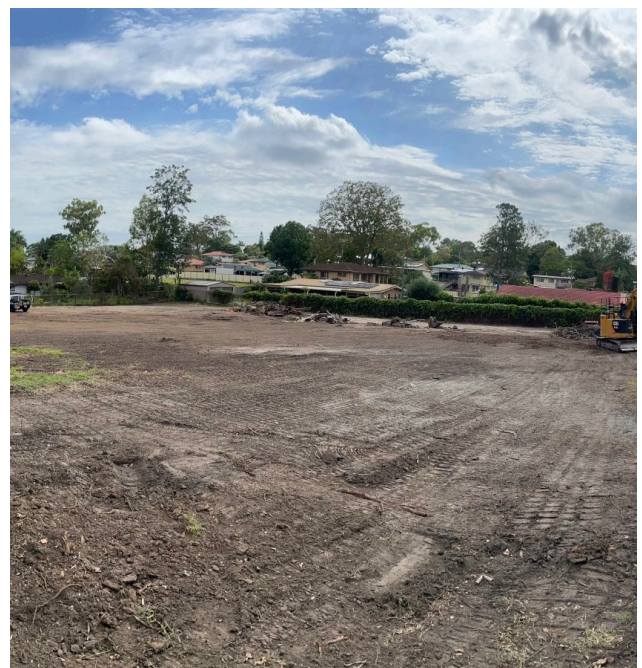
Clearing of the site has been completed
