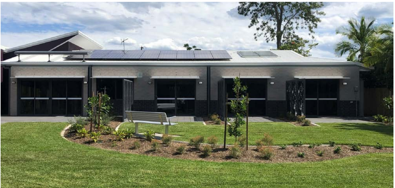
The NDIS high support home completed in November 2021
